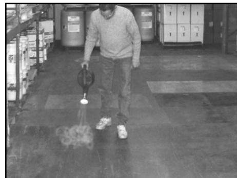
garden sprinkling can as uniformly as possible. Allow Etcher to work for 5 minutes. Scrub with low speed floor machine equipped with a grit brush. Pick up solution with a wet/dry vac or squeegee solution into floor drain. An automatic scrubber may also be used.
