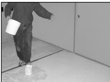
**Tip:** To achieve a uniform chip coverage, toss the chips upward over the freshly coated area.
